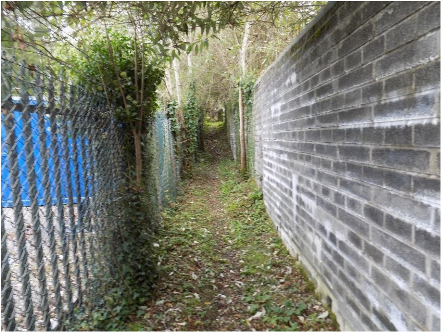
Figure 2-3.4: Down side approach to Wernddu Footpath Level Crossing
