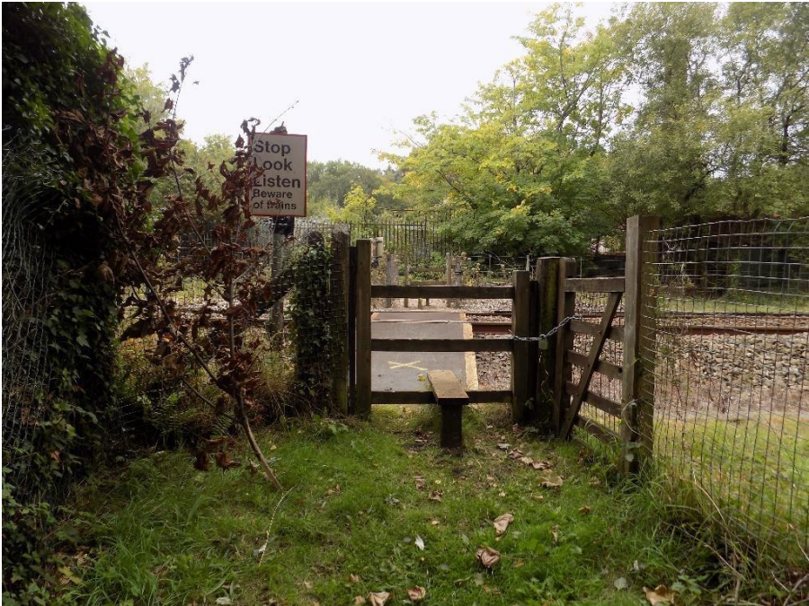
Figure 2-1.2: Current Arrangement at Wernddu Footpath Level Crossing (Down side)
