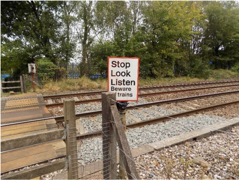
Figure 2-8.2.2: Signage on Down side
